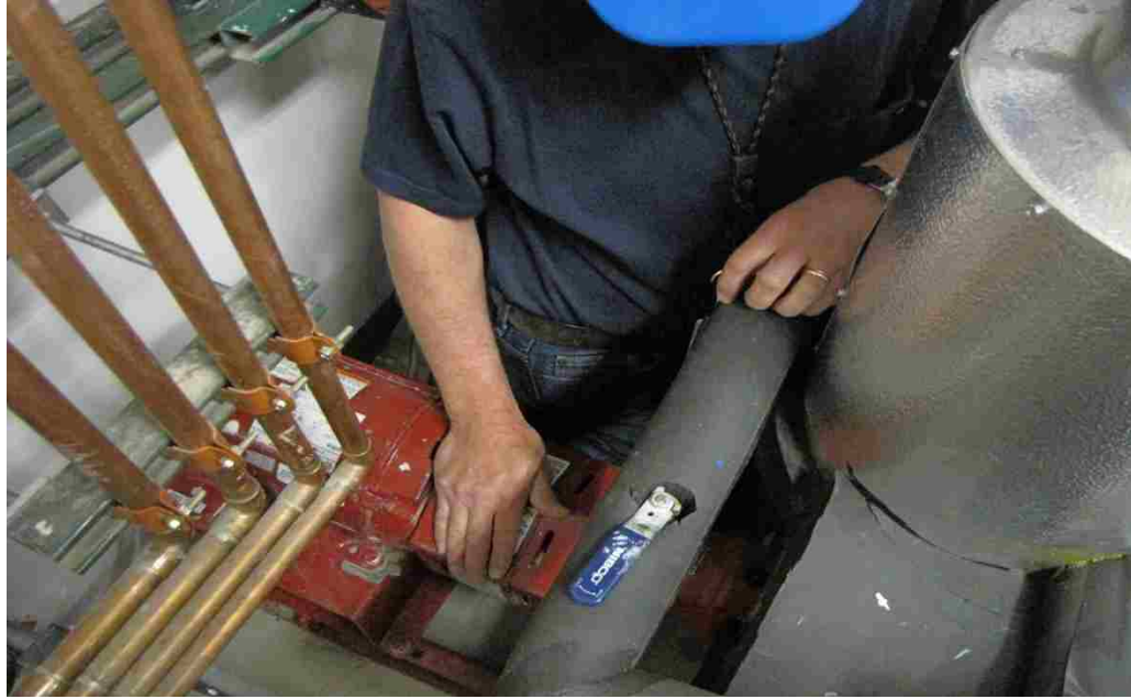
Figure 10: O&M worker performing maintenance work with limited space – Courtesy Birgitta Foster
